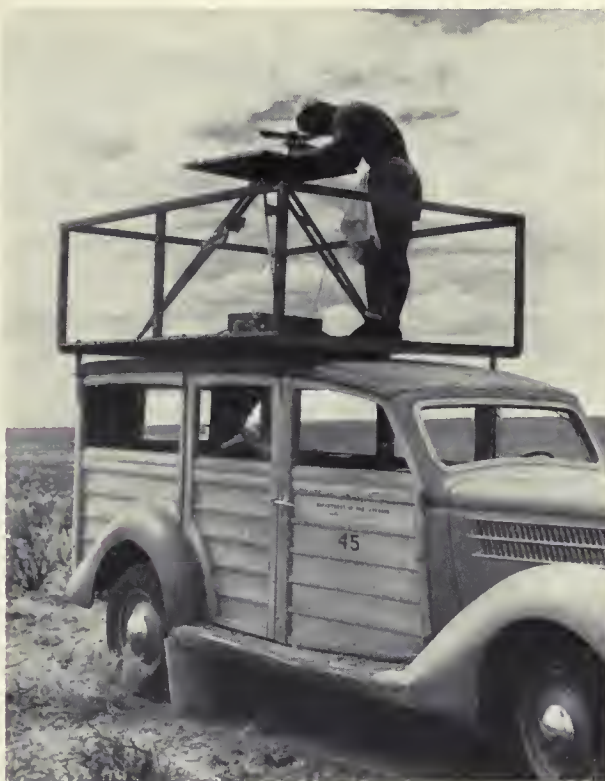
SURVEYING THE LAND in the heat of the August 1937 summer, using a platform on top of a station wagon to improve the topographic view of the Columbo Basin. Photographer unknown.
